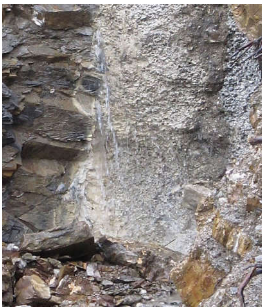
Figure 11. Run-off of drained water in the final section of the draining trench
