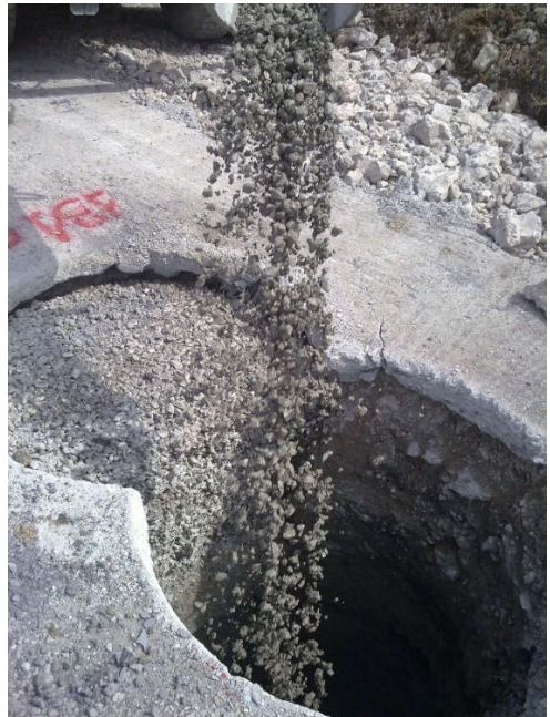
Figure 10. Construction of the secant draining pile (Phase B)
